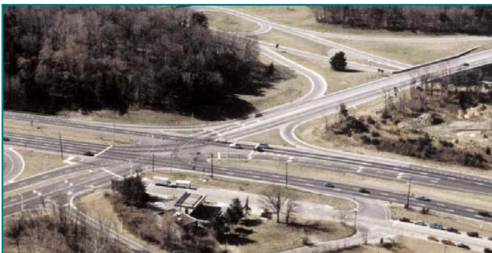
Aerial view of an existing intersection.
