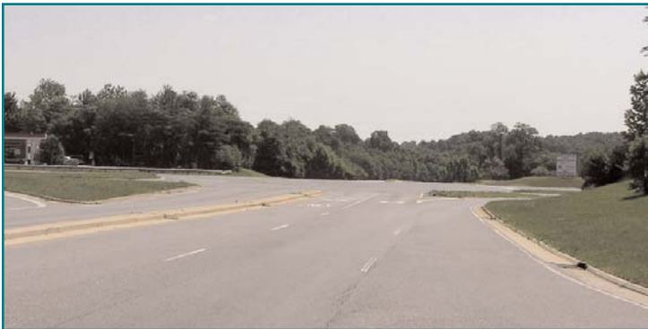
At-grade view of an existing intersection.
